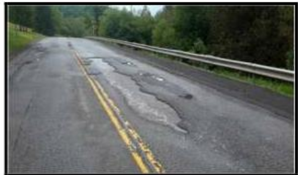
Pavement De-lamination.
